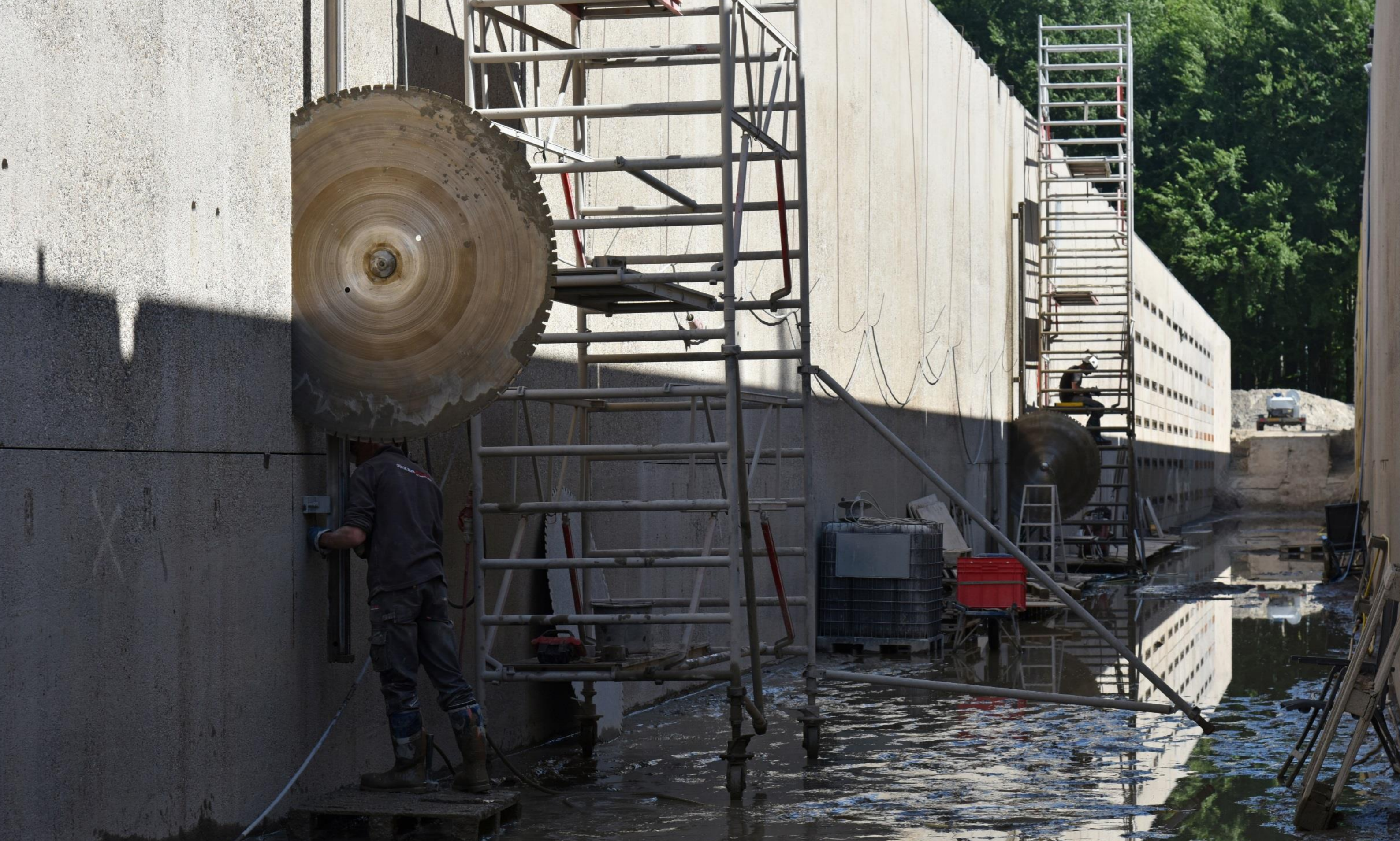
Cutting concrete
